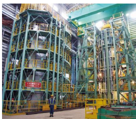
熱処理炉 Heat Treatment Furnace
