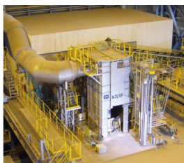
取鍋精錬炉 Ladle Refining Furnace
